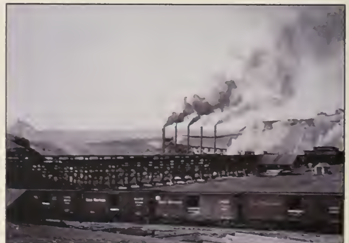
Cottonwood Coal Company, Stockett, Montana, showing tipple. (Montana Historical Society, Helena, used by permission).
